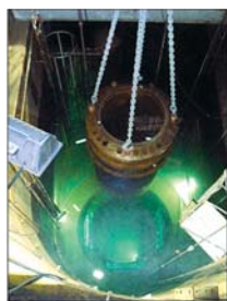
Removal of the Belgian BR3 reactor pressure vessel for further dismantling.
