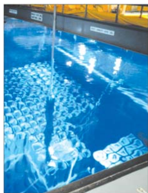
Typical spent nuclear fuel storage pool.
